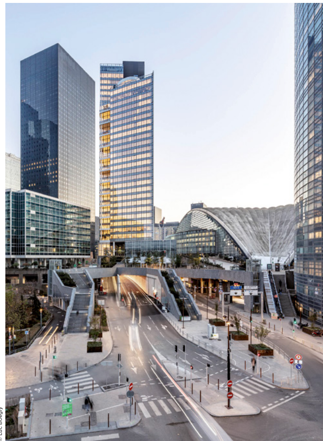
The Trinity Tower wasn't built on undeveloped land; it stands above the roads and motorways.
